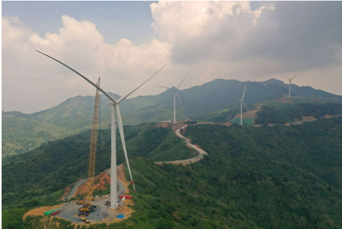
The 128 MW Tanay Wind Project in Rizal, one of the two assets covered by A Brown's ₱2.3 billion investment, expected to commence commercial operations later this year.
